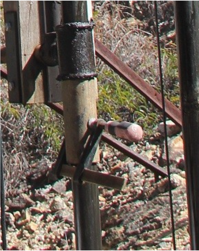
CLAMPS STOP FRAME FROM SLIDING DOWN
